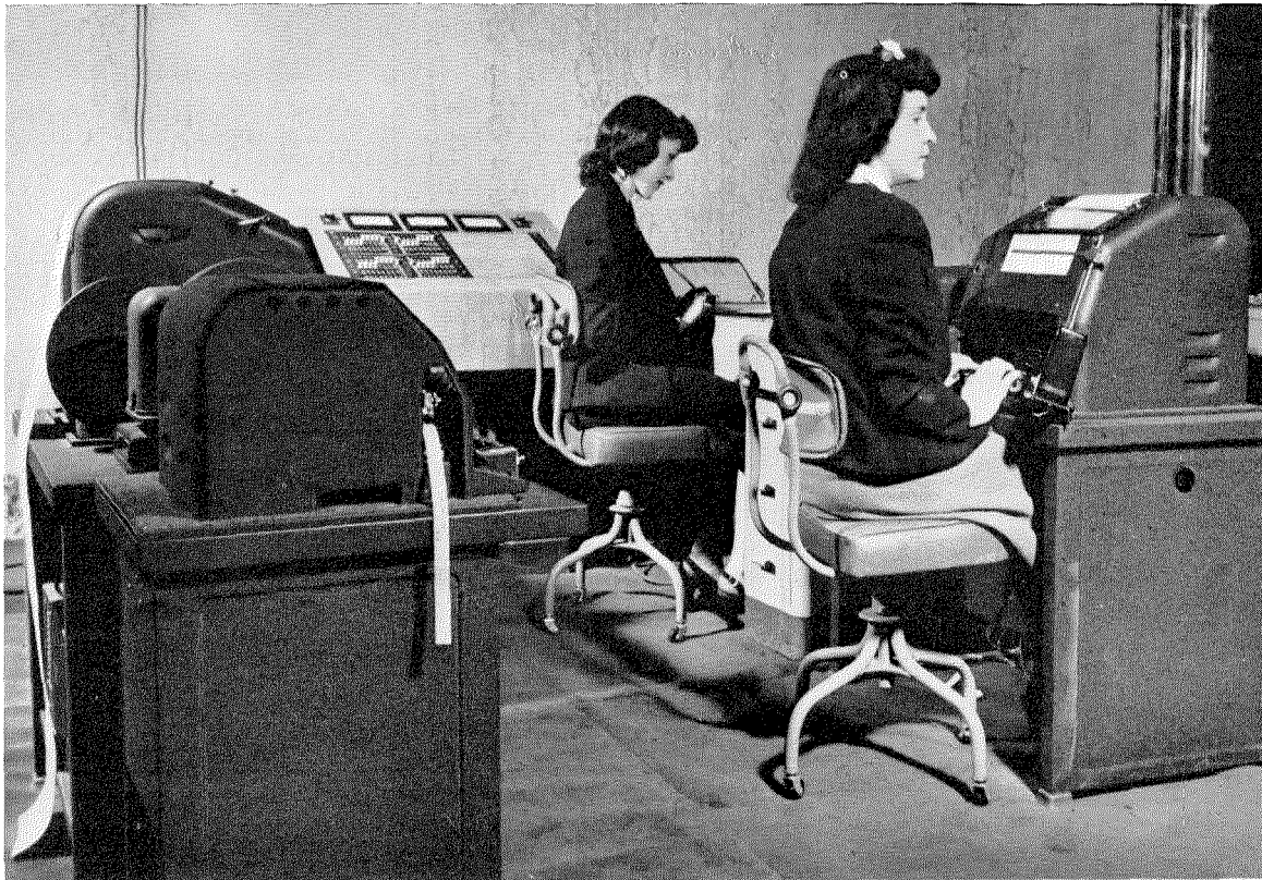
Intelex central office. The operator in the foreground is using the monitor teleprinter. The logging teleprinter and the teleprinter broadcast transmitter appear in the left foreground. At the back are the meters and jack panels for monitoring and adjusting the operation of the Intelex equipment.
