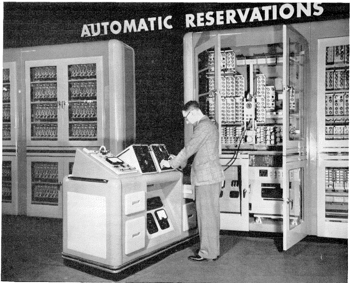
Engineer checking Intelex operation by means of equipment on test-set console. The racks in back of the console include switches, called the ledgers, for the storage of reservation information.
